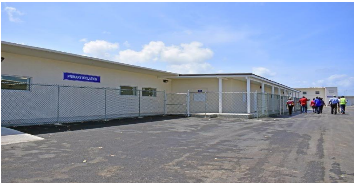
Figure 1. Harrison Point Facility
